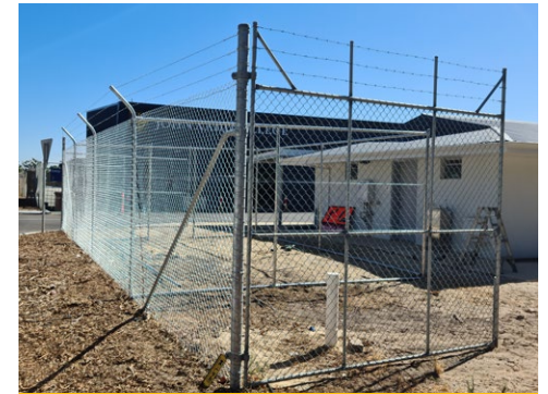
Galvanised Chainwire Fencing with Barb Wire
