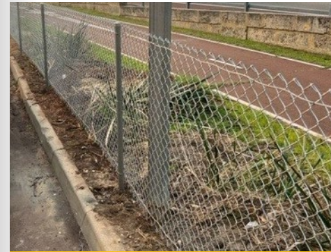
Galvanised Chainwire Fencing with Galvanised Posts
