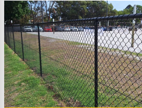
Black Chainwire Fencing with Powder Coated Posts & Rails
