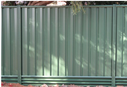
Colorbond Fencing with Retaining Plinth
