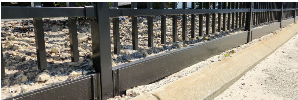
Garrison Security Fencing - with Retaining Plinth
