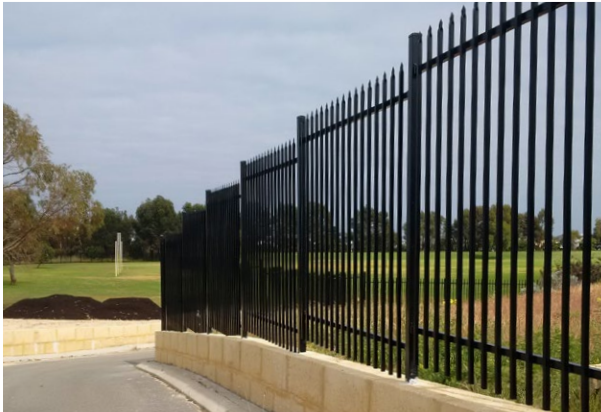
Garrison Security Fencing - Installed on Limestone Wall
