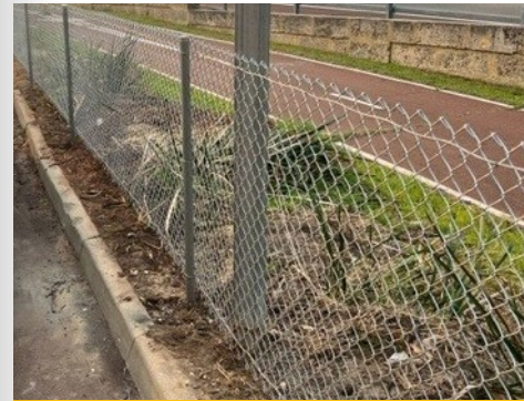
Galvanised Chainwire Fencing with Galvanised Posts
